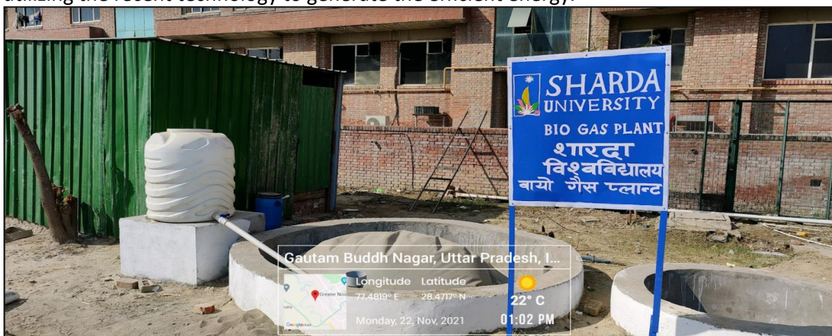
(Biogas Plant near Block 7)
