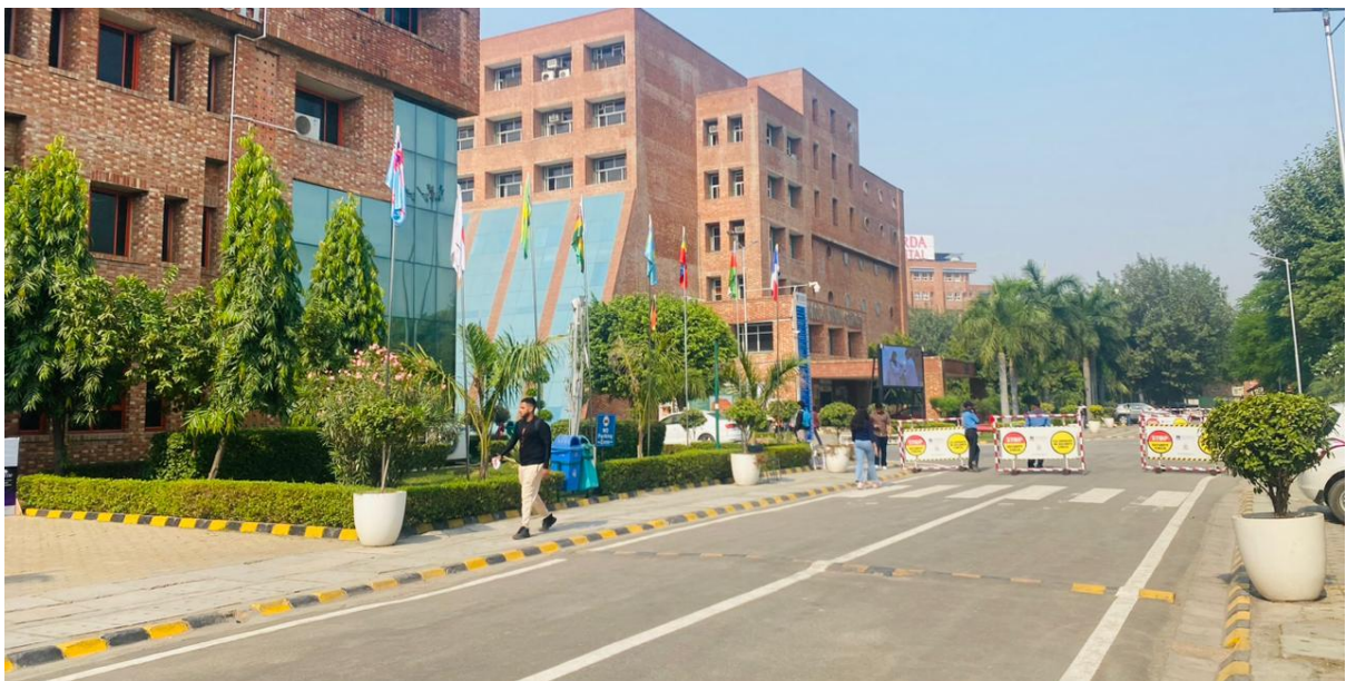
Fig 48 Traffic barriers to restrict vehicular movement
