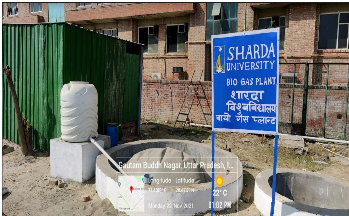
Fig.14. Biogas Plant near Block 7 (Sharda University)
